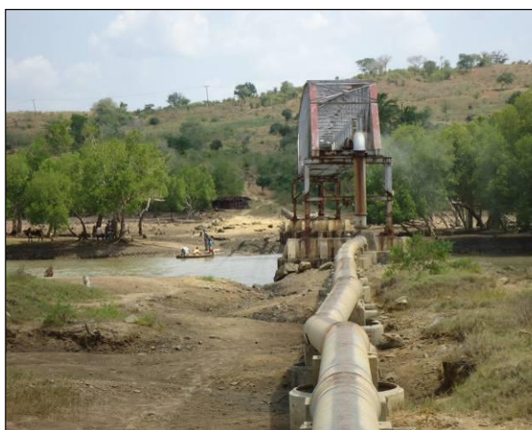
Marere Pipeline crossing towards Mazeras Tanks
