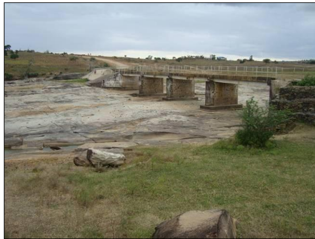
Bridge over Mwache (Mazeras – Kinango)
